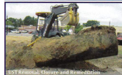
UST Removal, Closure and Remediation
