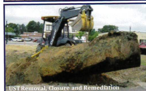
UST Removal, Closure and Remediation
