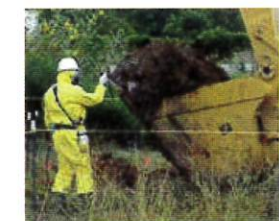
Contaminated Soil Removal
